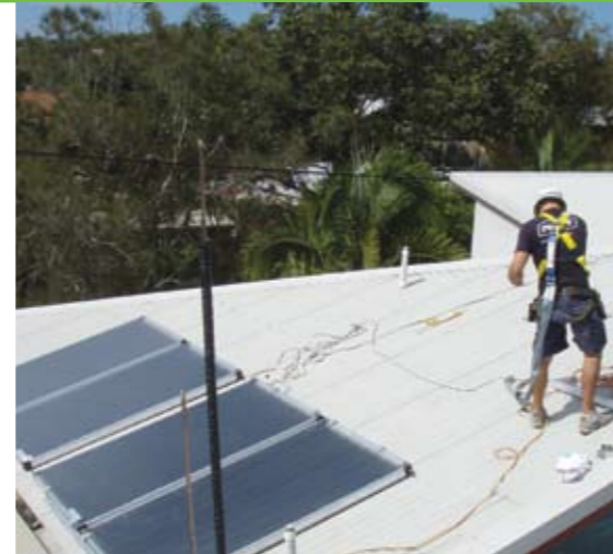
Installing solar panels at Byron Bay YHA
