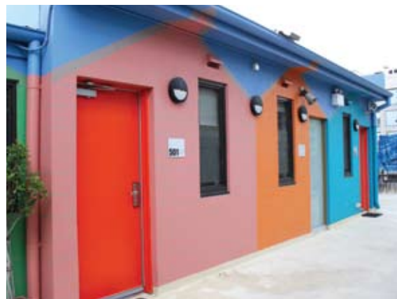
Extra rooms were added on the rooftop at Melbourne Central YHA
