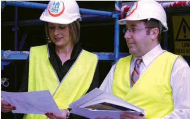
Kristina Kenneally (as NSW Planning Minister) and Ross Lardner (Hostel Manager) on construction site of Sydney Harbour YHA
